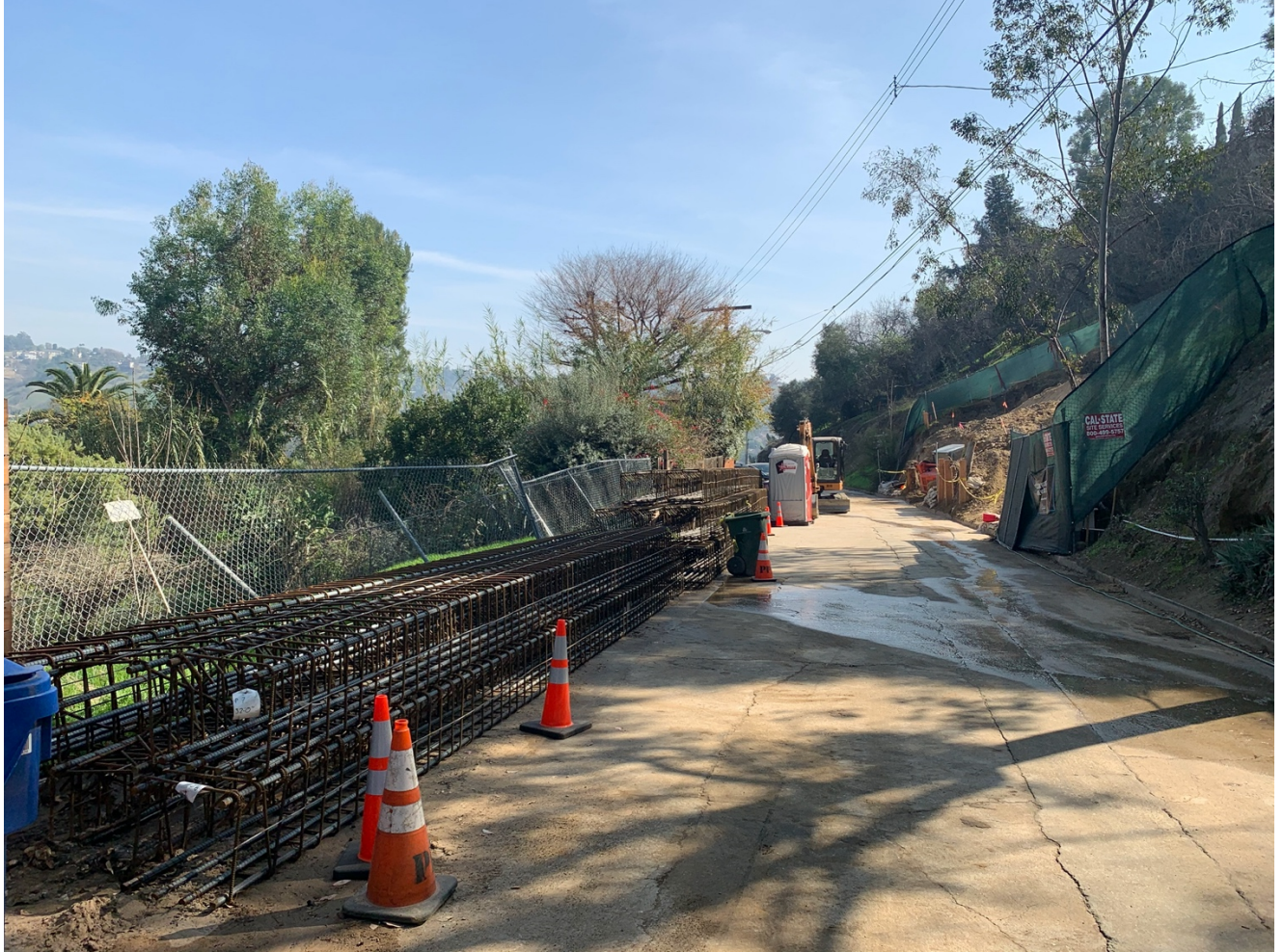
Construction materials stored on the street opposite the construction site and down the street with no night-time safety lights and no street permit displayed. Porta-potty on the roadway. Construction equipment parked on the roadway and fencing in the road. Taken on a "paved" portion of Glenalbyn.
